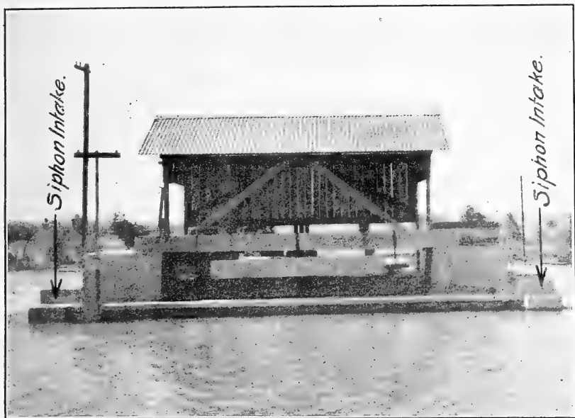
FIG. 1.—AUTOMATICALLY OPERATED GATE WITH SIPHON SPILLWAY ON EACH END. Located on main distributing canal, South San Joaquin Irrigation District, near Ripon, Calif.
